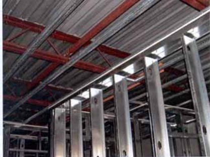
Floor joists, hat track and light gauge steel framing
