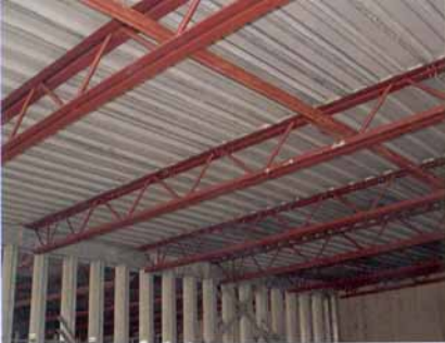
Floor joists as seen from below
