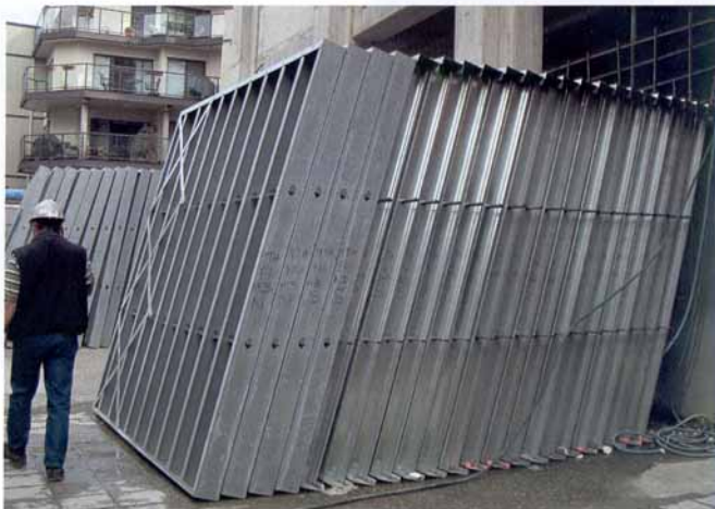
Prefabricated steel stud framework, manufactured to contractor specifications by Steeler Inc.
